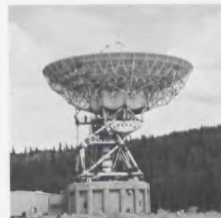
The large "dish" antenna is 98 feet in diameter. It sends and receives communications via satellite stationed in orbit 22,300 miles above mid-Pacific.
