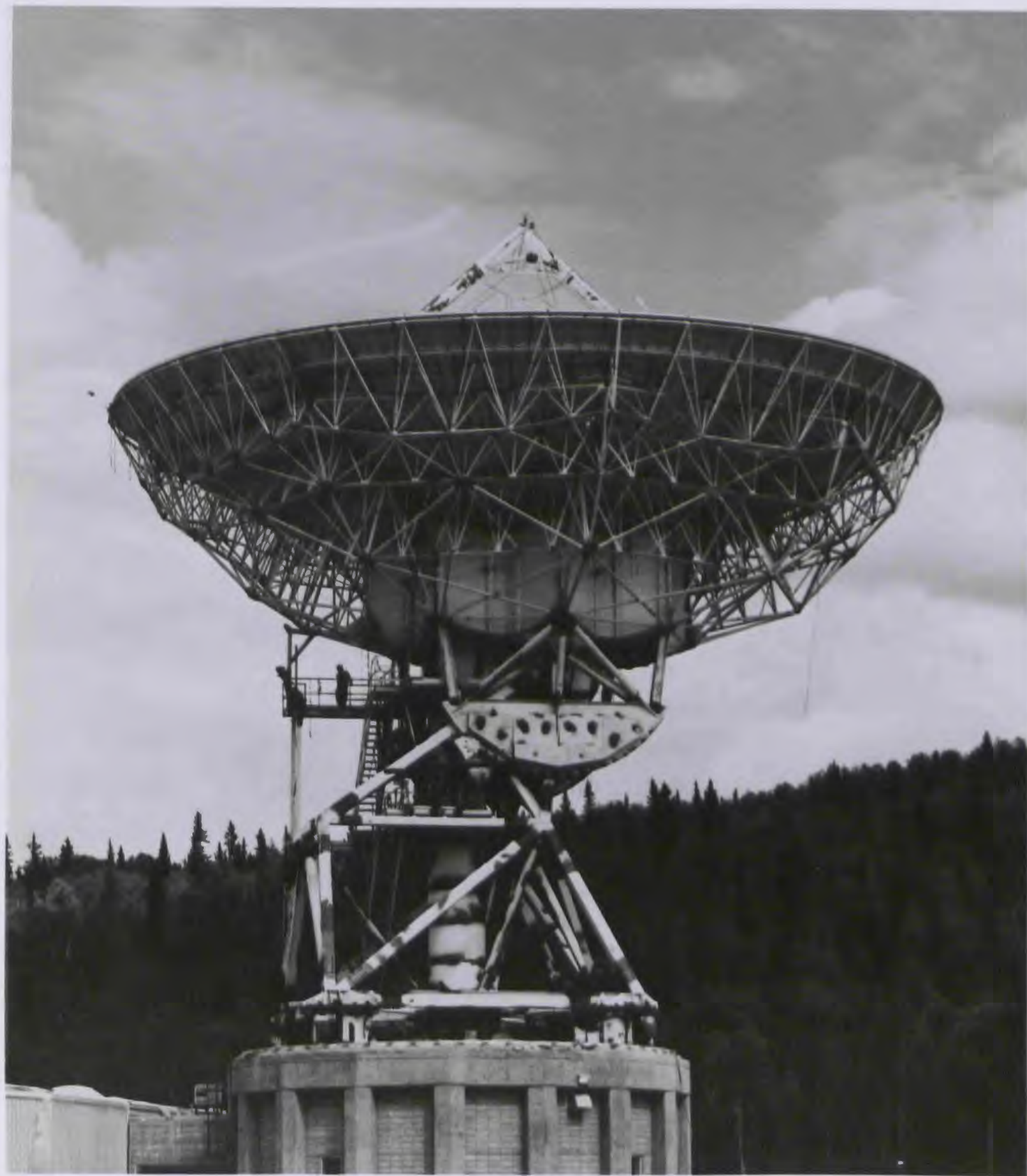
The Bartlett earth station near Talkeetna, Alaska, newest and most northern in today's global satellite system, is equipped with a "dish" antenna 98.4 feet (30 meters) in diameter. The station can send and receive all forms of commercial communications via satellite: telephone, telegraph, facsimile, data and television.
