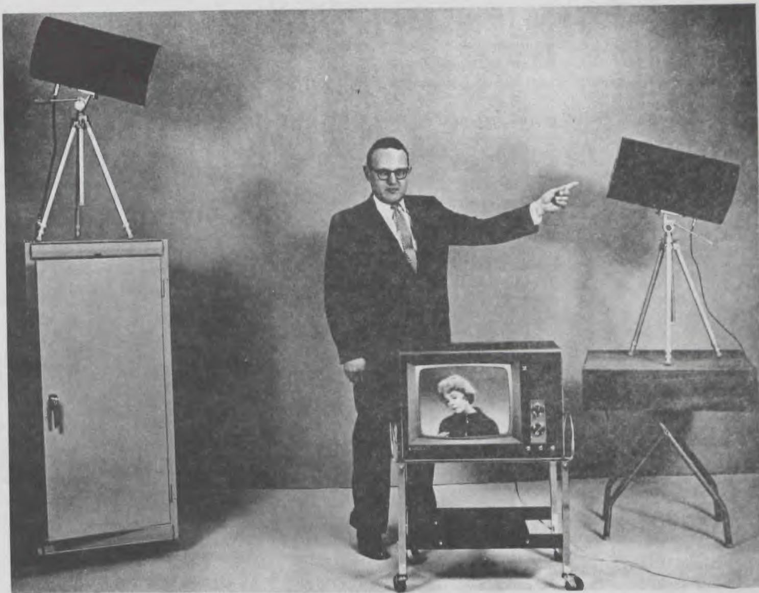
Figure 2. QUASI-LASER LINK SYSTEM IN EXPERIMENTAL OPERATION (with TV pix)
