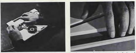
Developed by the AEC's Argonne National Laboratory, this instrument is designed to reproduce symbols in the Braille alphabet that have been recorded on ordinary magnetic tape — thereby increasing the volume and reducing the cost of Braille literature.
