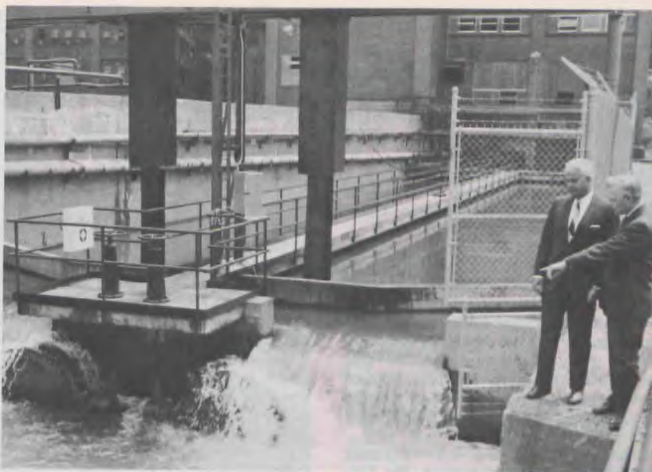
Water processed by Goodyear's new $750,000 environmental control facility is inspected by Board Chairman Russell DeYoung (left) and T. F. Minter, director of manufacturing services. A system of screens, settling basins, pumps and oil skimmers brings the Little Cuyahoga River up to state standards at this point where it leaves the company's manufacturing complex in Akron, Ohio.
