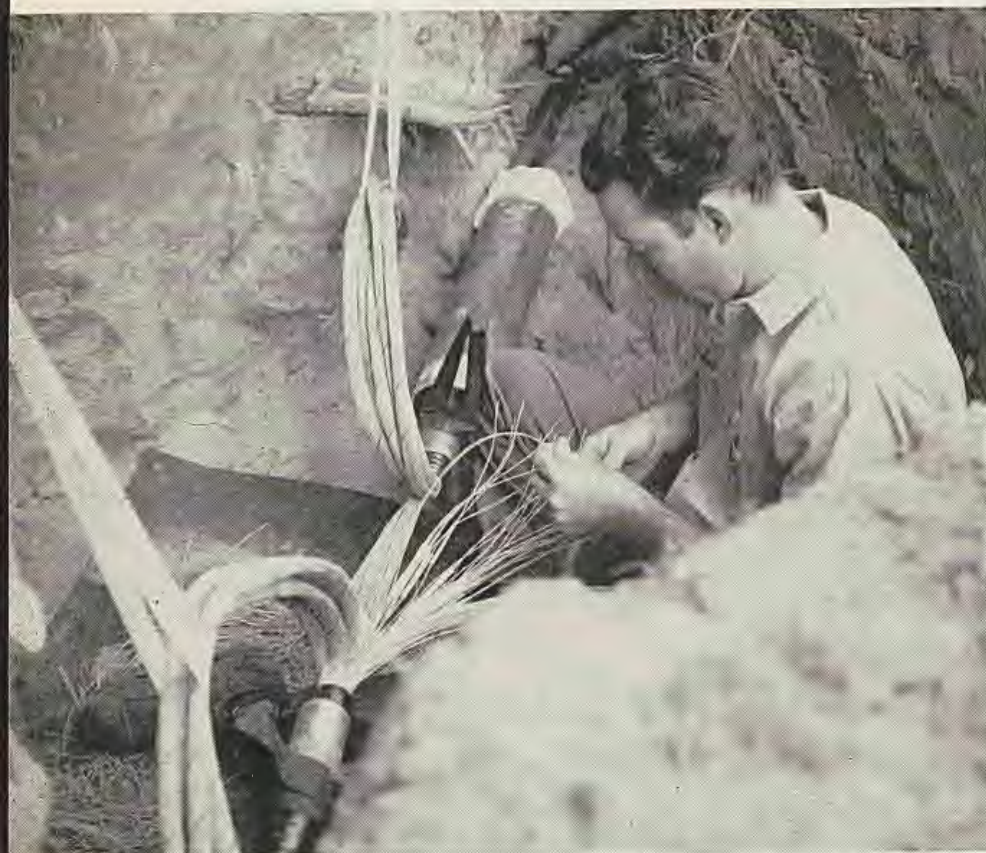
A LOT OF cable splicing is done when a company grows as quickly as Winter Park Tel.
