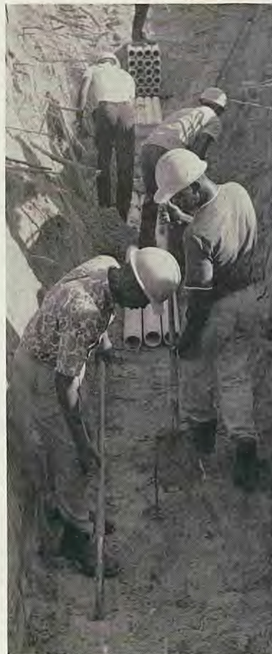
WHEN underground conduit is installed, WPT provides enough ducts to care for projected future requirements.
