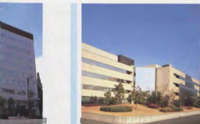
ITJ Tokyo Telecom Center
