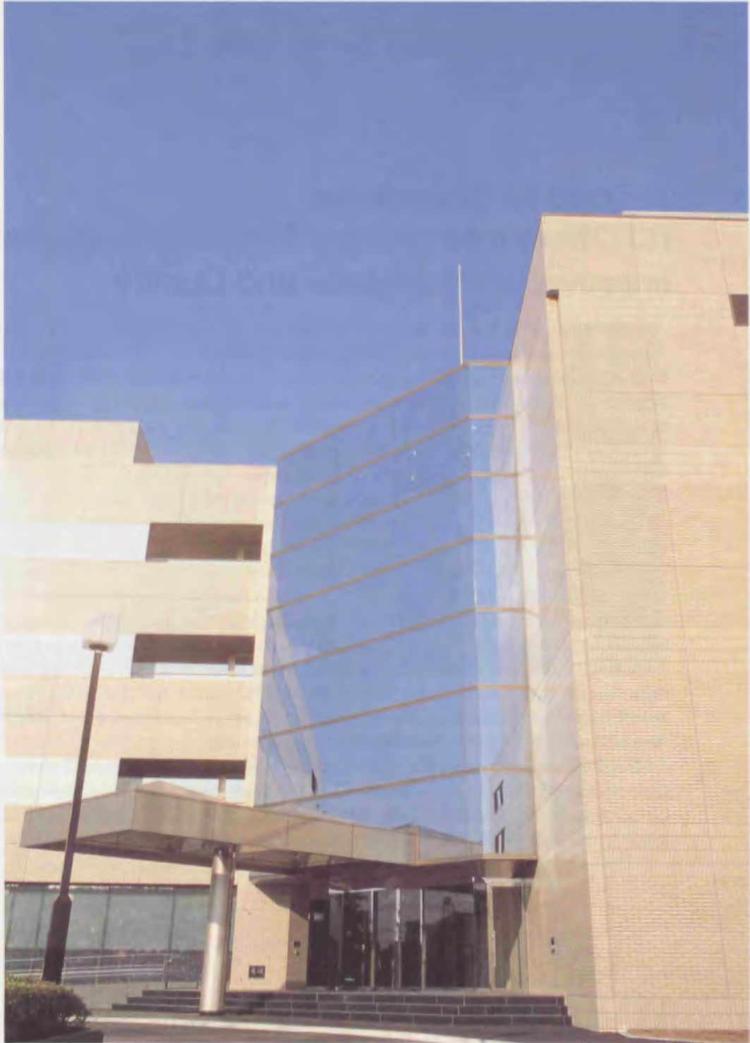
ITJ Tokyo Telecom Center
