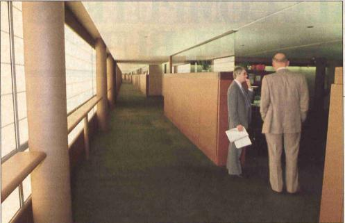
The fiberglass wall at left allows in daylight to illuminate the hall.
