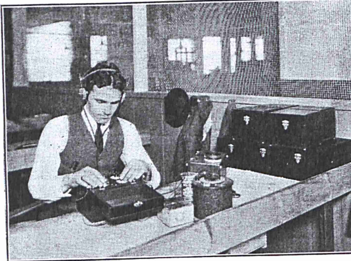
FIG. 9 FINAL TEST ON AERIOLA JUNIORS The test is for wave length, oscillation, and audibility.
