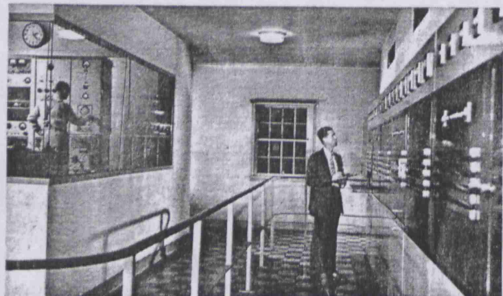
KDKA's Chief Engineer, T. C. Kenney, records data from dials at the transmitter station. Behind these metal walls are wires, vacuum tubes, electrical condensers, coils, switches, relays and much other complex apparatus representing years of research.
