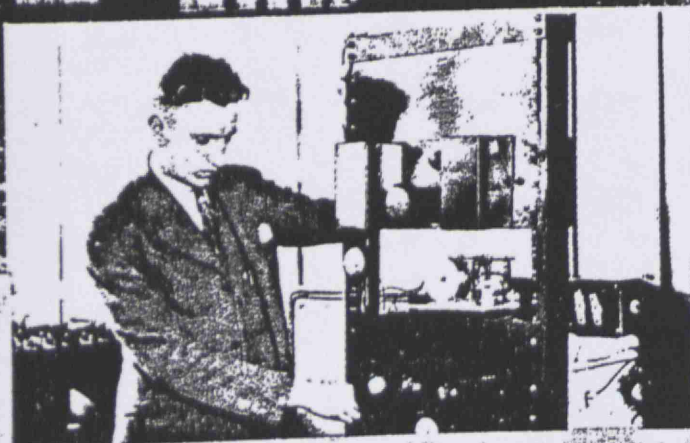
Lester J. Wolf, currently in DEP Radar Projects at the Moorestown plant, is shown with a developmental quartz crystal frequency standard at Westinghouse, 1928-29.
