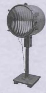
Fig. 63-Airport Landing Floodlight (Closed).
